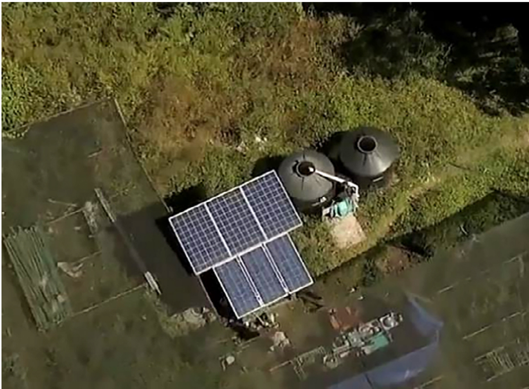
Electrification pumping system for productive processes in isolated communities and rural areas in San Felipe Usila, Oaxaca, implemented in June 2018. (FOTEASE, 2022)
